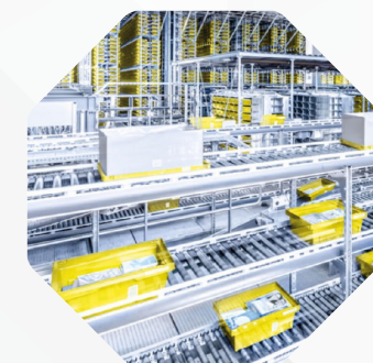
Material Handling Logistic
